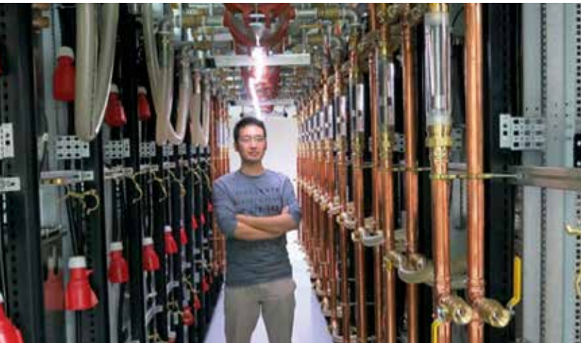
Example of a modern bitcoin mine, ASCIMiner, in Hongkong's Kwai Chung. The cooling installations are on the roof of the building.
